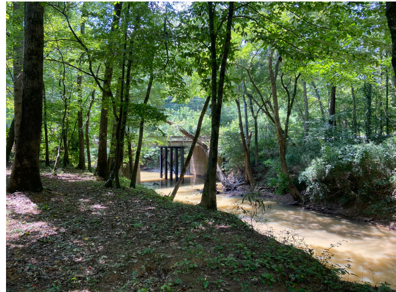
9. Looking toward Waxhaw-Marvin Bridge from trail (Segment 5)
