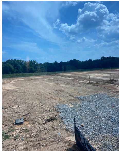
13. Encore neighborhood under development, looking toward future trail area (Segment 7)
