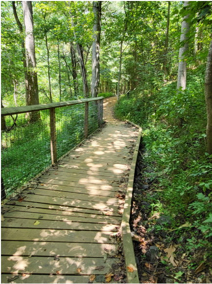
1. Existing boardwalk (Segment 1)
