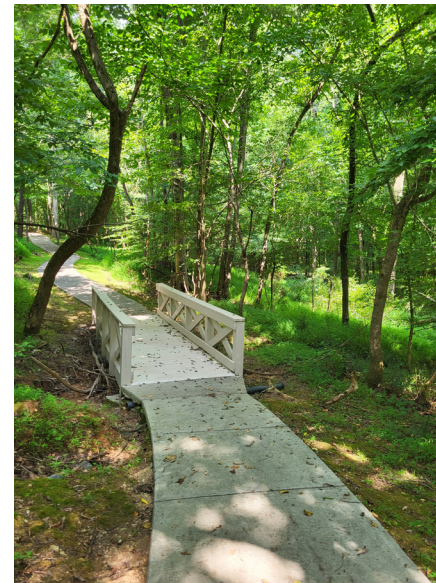
14. Bridge on existing Lawson Walking Path (Segment 9)
